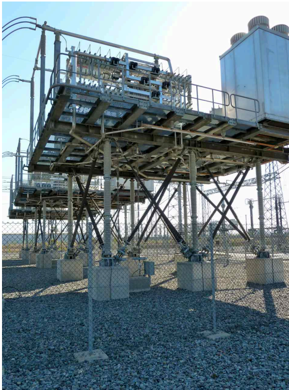
Capacitor bank without damage
